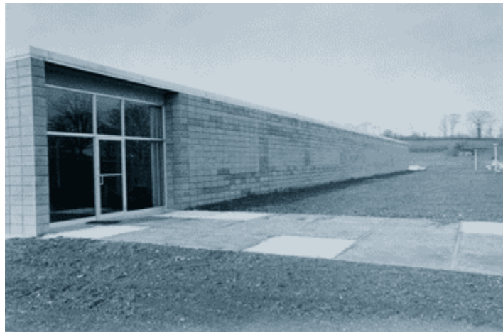
In 1966 DSI moved into a new factory and corporate offices located in Poestenkill, New York. This photo was taken just after completion of the new building.
